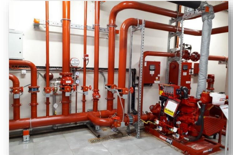
Fire Pump Station
