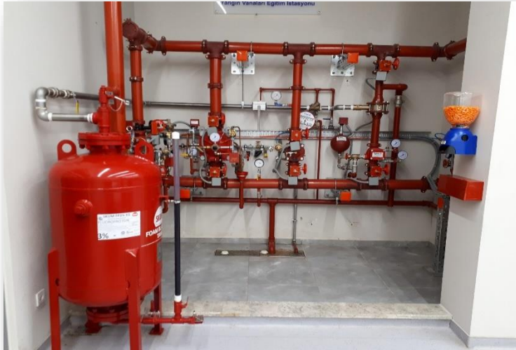
Alarm Valve Station
